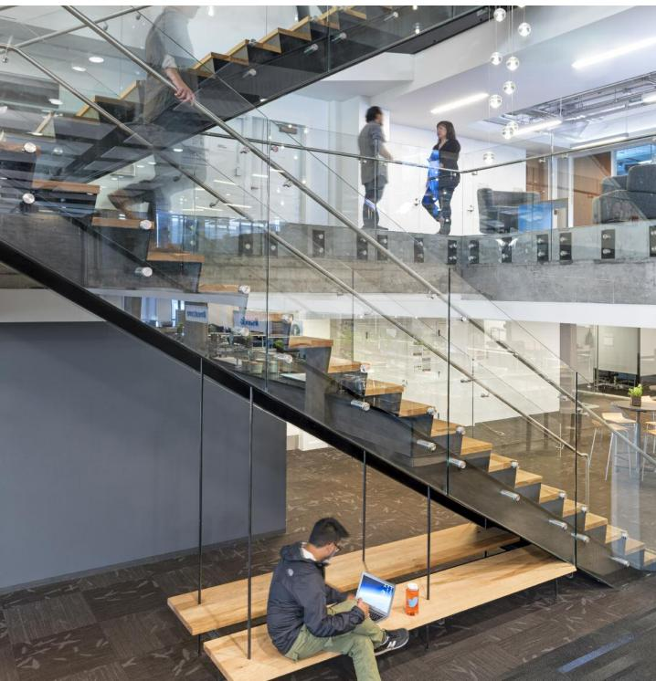
Optik *POD*™ creates the impression of complete transparency with structural glass panels. The Optik POD system provides discreet structural brackets to support the glass guardrail and are available in a variety of designs, which can be either round, elliptical or rectangular to suit you project needs. All fasteners are completely hidden from view providing clean lines from elegantly simple shapes. Available glass thickness is ½" or ¾".
